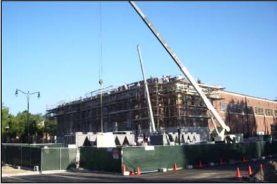
Once the entire building was in the dry, we used cranes on both corners of the addition to install the limestone and brick veneer. We were able to systematically restore thousands of square feet of existing limestone and brick to blend the existing and new portions of the building together.
