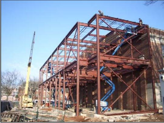
Concurrent with the interior retrofit, the exterior was receiving a complete update, including an addition to the south end of the building. The second floor addition was specifically designed to accommodate the mechanical and electrical equipment for the entire 50,000 square foot building. In order to maintain our completion date, once this part of the building was in the dry, 50 ton cranes were used to drop the mechanical units through 16' by 16' roof hatches.
