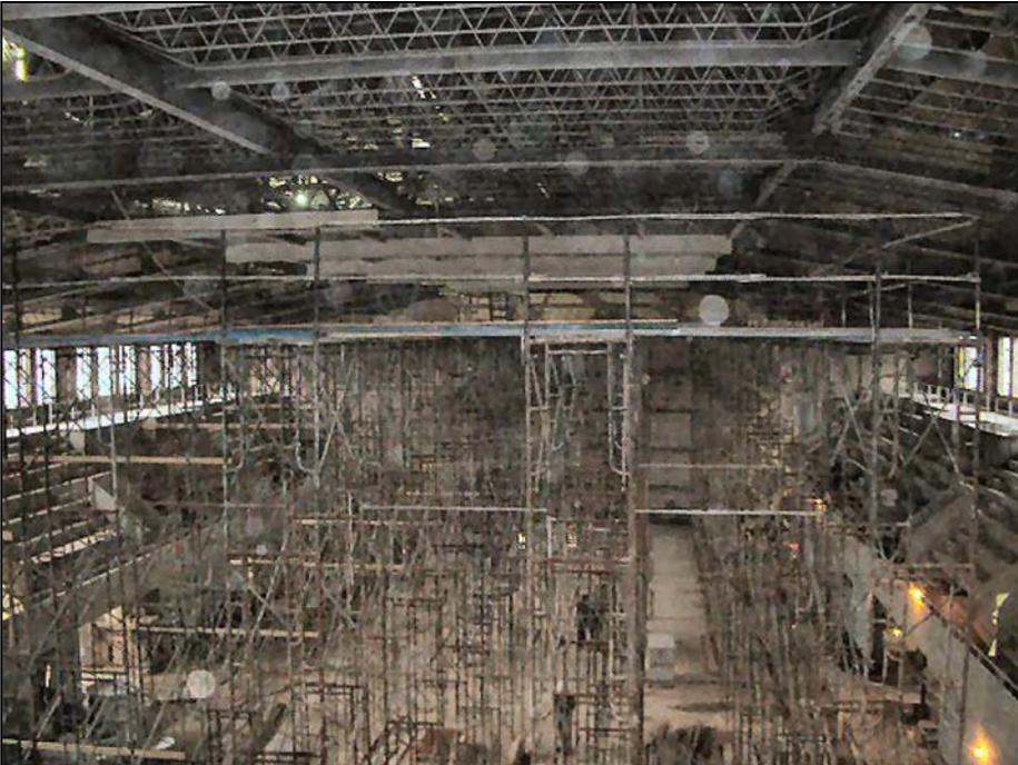
Once the floor was complete, we installed 15,000 square feet of scaffolding ranging from 30' to 50' in height; this enabled installation of the overhead electrical, mechanical, stage rigging and AV systems. Concurrent with this work, we rehabilitated a 1939 era skylight system and installed a curvilinear ceiling of acoustical plaster. Prior to dismantling the scaffolding, all overhead fixtures were installed, trimmed out and dust wrapped in preparation for final use.
