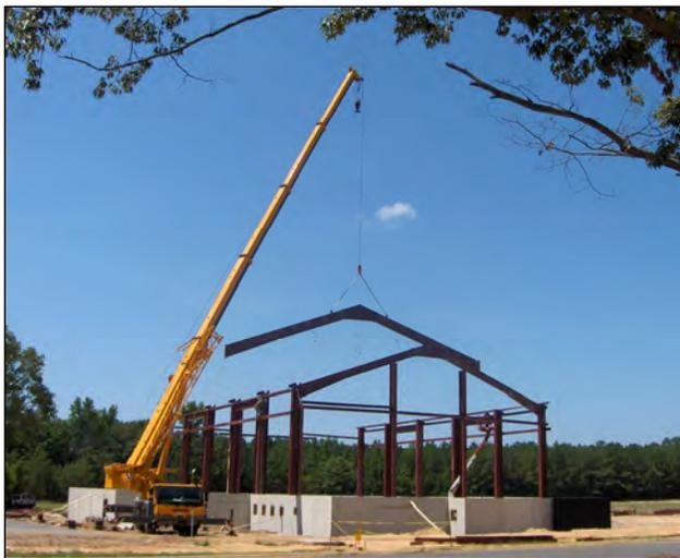
We installed a pre-engineered building system with bearing in the basement that extended through the first floor, all the way to the roof. After the roof was installed, we placed a versa deck system on top of the classrooms to create the first floor platform. Smaller portions of the building were constructed with steel studs and steel trusses. In the end, we used each system where it made economic sense and allowed a rapid schedule to get the building in the dry.
